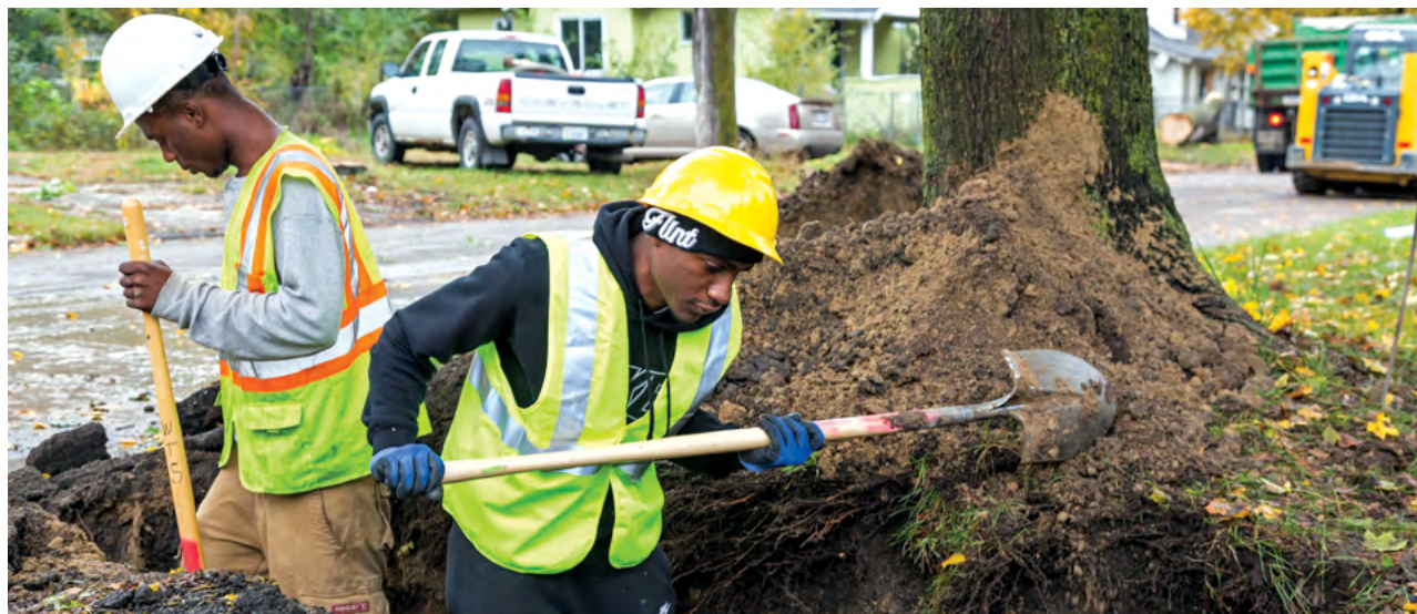
Workers replace water service lines in Flint.
